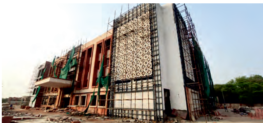
Construction work at new office building
